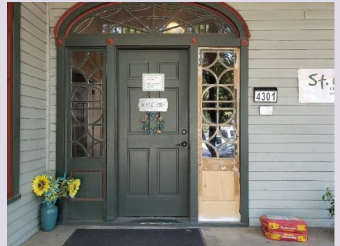
Replaced side glass panel for front door.
