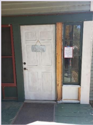
Replaced solid wood back door and kick panel to right.
